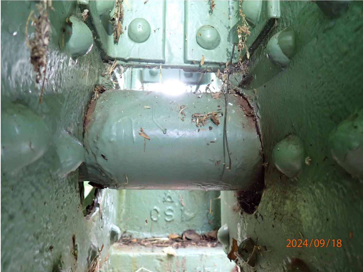
Pratt Truss 1, L0 bearing north side of pin
